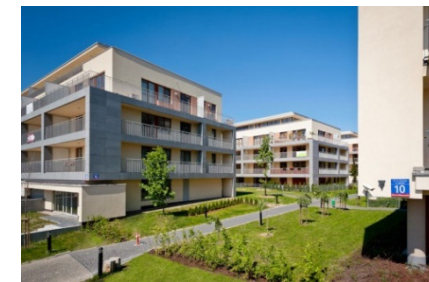
Ostoja-Wilanów (stage 6, building C3). Date of delivery: October 2011. No. of units: 262 apartments (16,278 sq. m). 10 commercial units (kindergarden).
