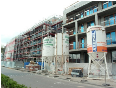
Ostoja-Wilanów, Warsaw, (stage 8, building B2).
