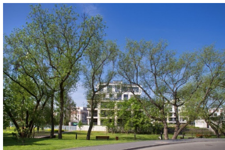
Ostoja-Wilanów (stage 7, building C4). Date of delivery: December 2013. No. of units: 324 apartments (19,688 sq. m).
